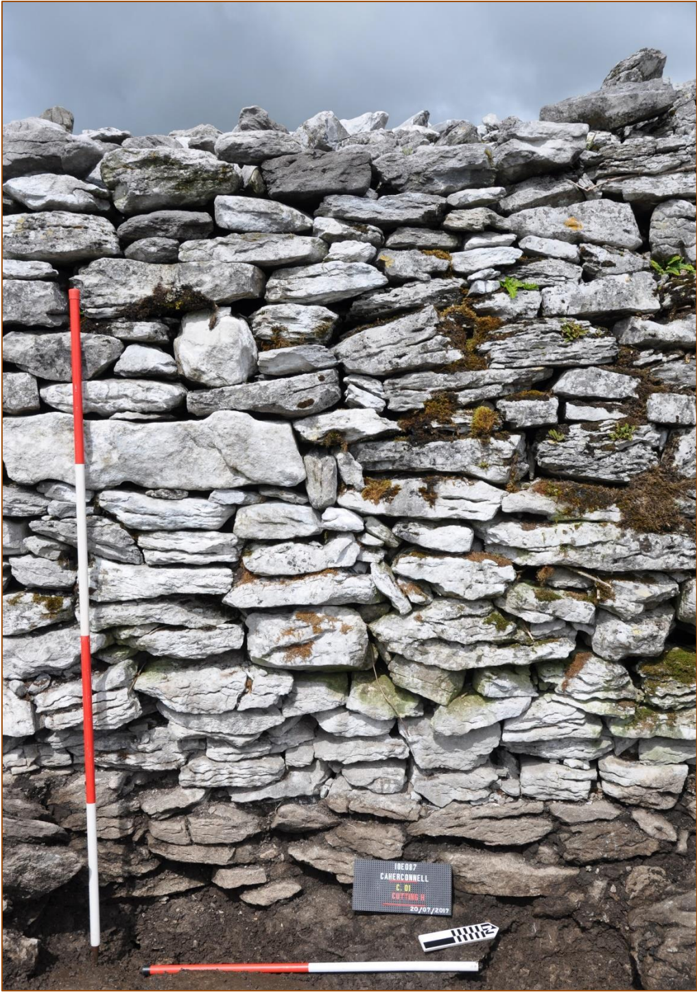
Fig. 16 Cashel wall in Cutting H. Scales 2m and 1m.
