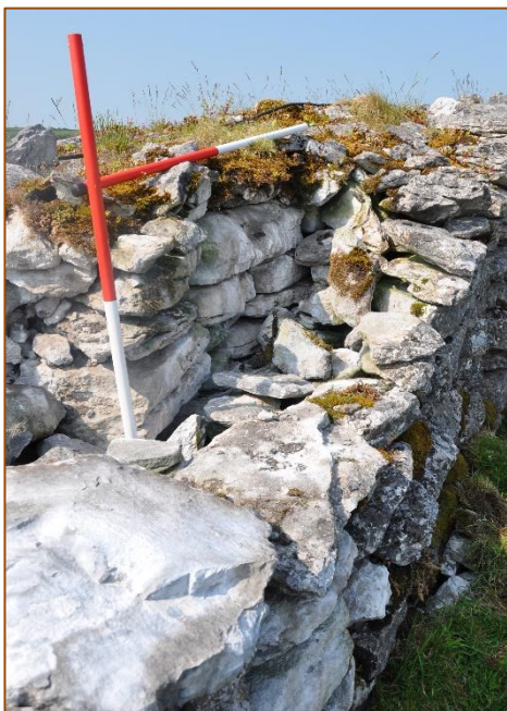
Fig. 15 Extra 'skin' added to internal face of cashel wall.
